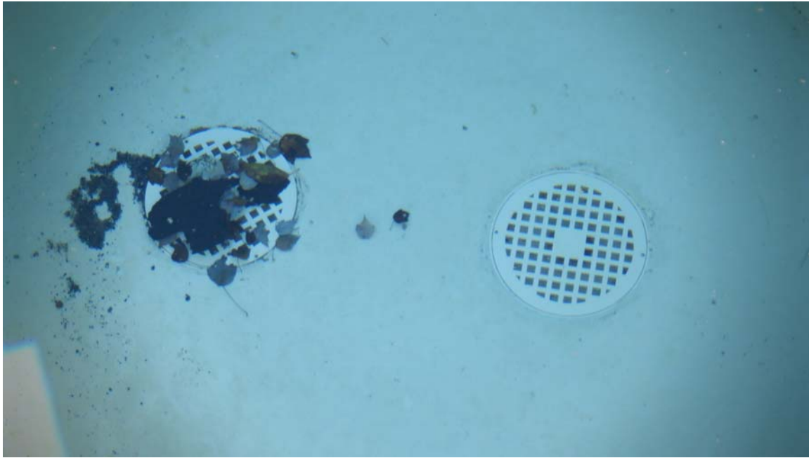
Picture 9 - Spa Drain Covers not VGB/Anti-Entrapment Compliant
