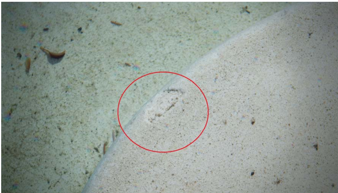
Picture 2 - Chipped plaster on steps.
