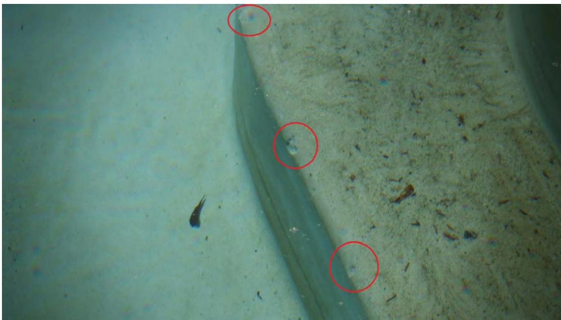
Picture 2 - Chipped plaster on steps.
