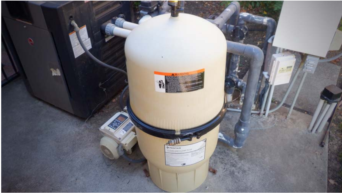
Picture 11 - Pentair Clean and Clear Plus (CCP) 420 Cartridge Filter
