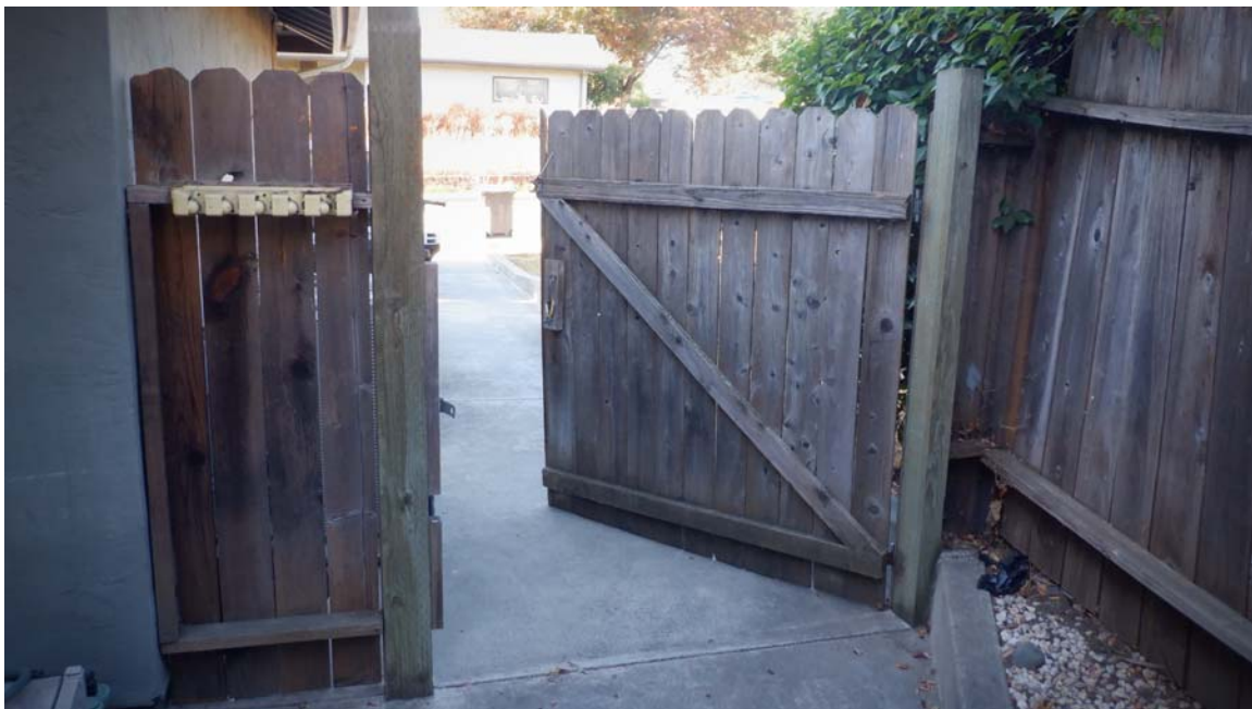
Picture 26 - Backyard access gate is not Self-Closing/Self-Latching.
