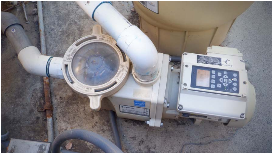
Picture 12 - Pentair Intelliflo VS (variable speed) Pump.
