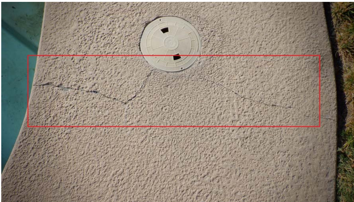
Picture 6 - Crack on concrete deck.
