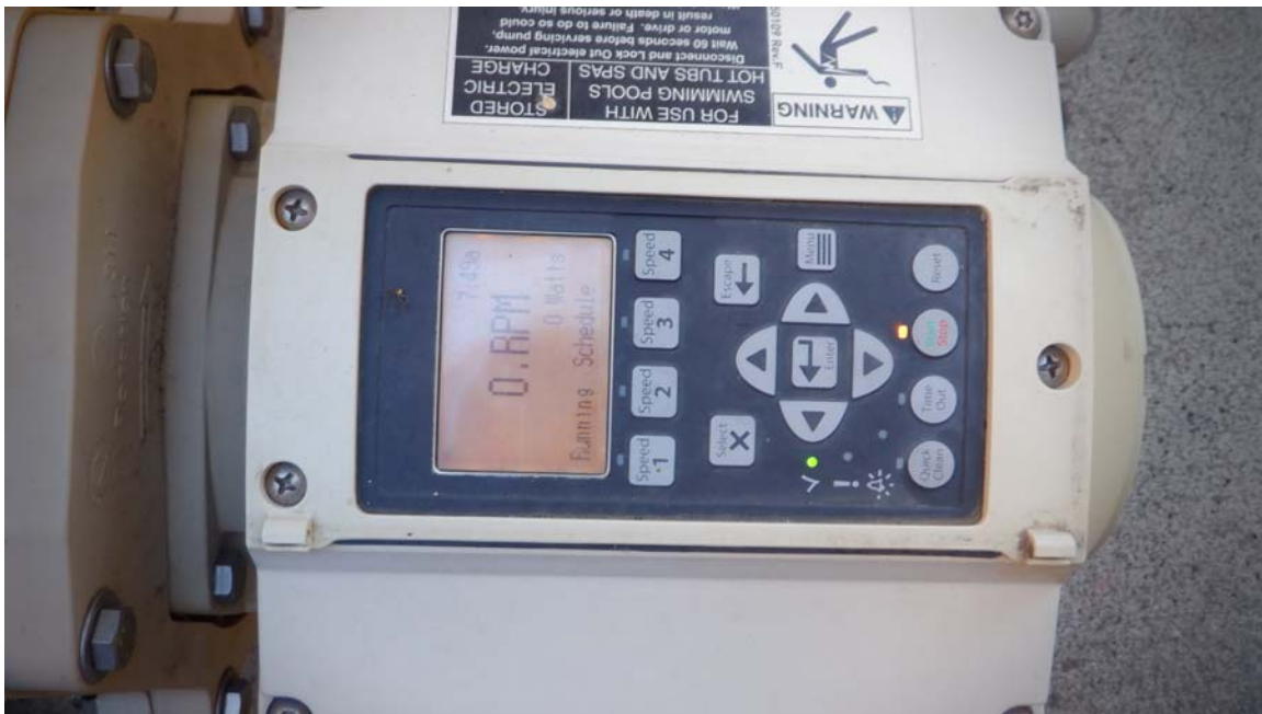
Picture 20 - Controller on pump for filter system
