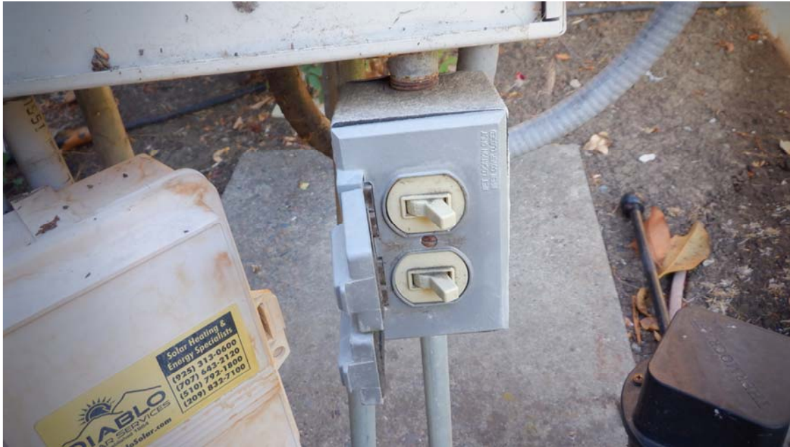
Picture 20 - Controller on pump for filter system
