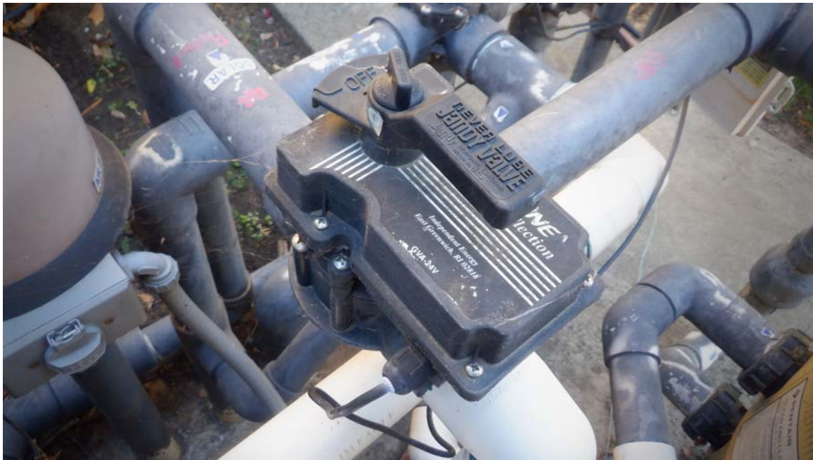
Picture 24 - Valve Actuator for Solar Operation.
