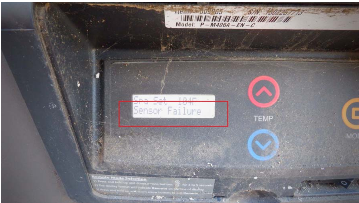
Picture 22 - Heater display reads "Sensor Failure"
